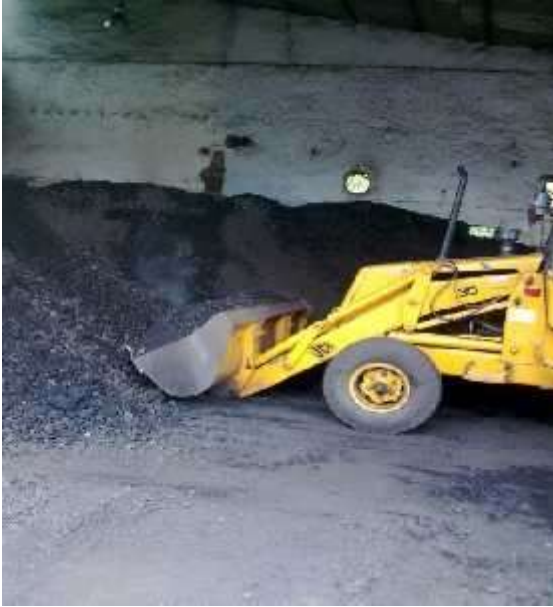
Lifting of Fuel Coal for Charging with JCB from Fuel storage shed.
