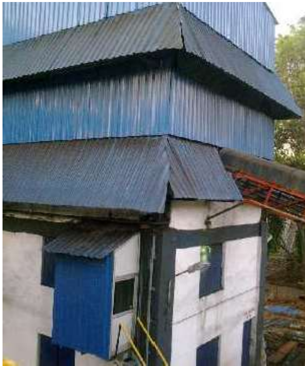
Coal Crusher House
